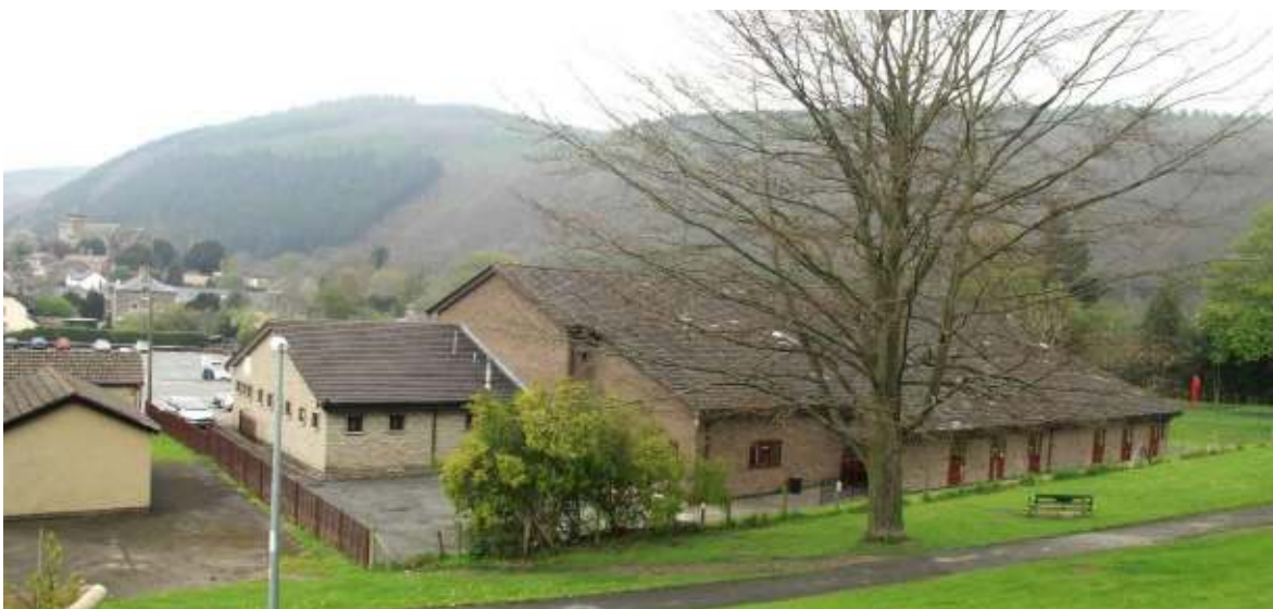
The rear of the Community Centre from the adjoining park
