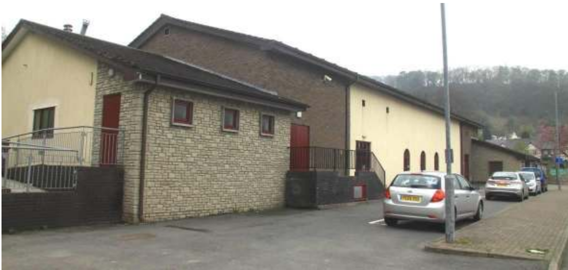
Above - two views from the public car park at the front
